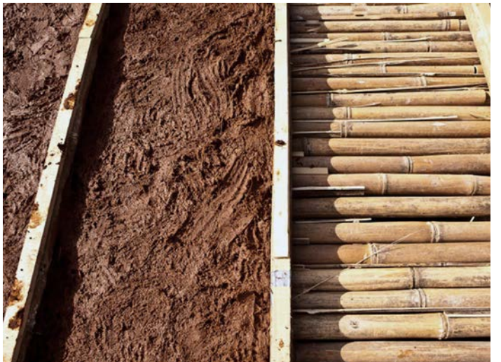
Layer of clay on bamboo ceiling in the dormitories
