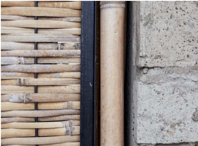
Bamboo door and column, wall made of local, natural stone
